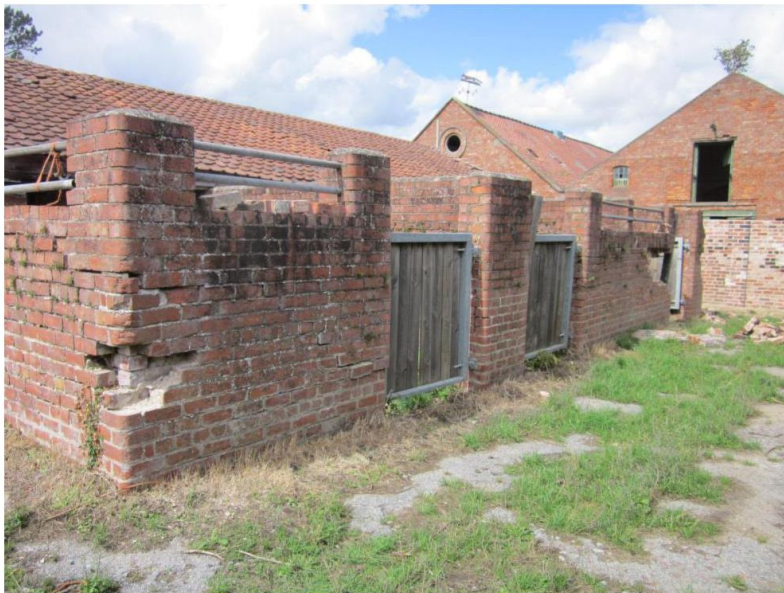
Fig 21 Building 5 East elevation of pigsties
