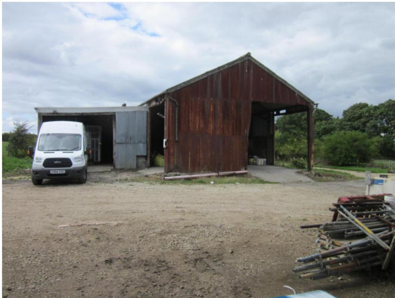
Fig 27 C20 steel-framed north-west shed
