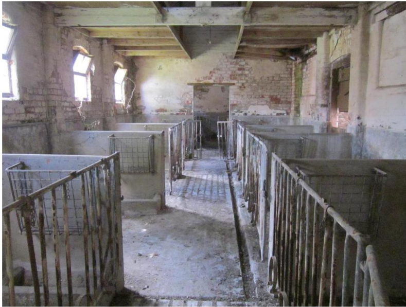
Fig 18 Building 4 East range interior
