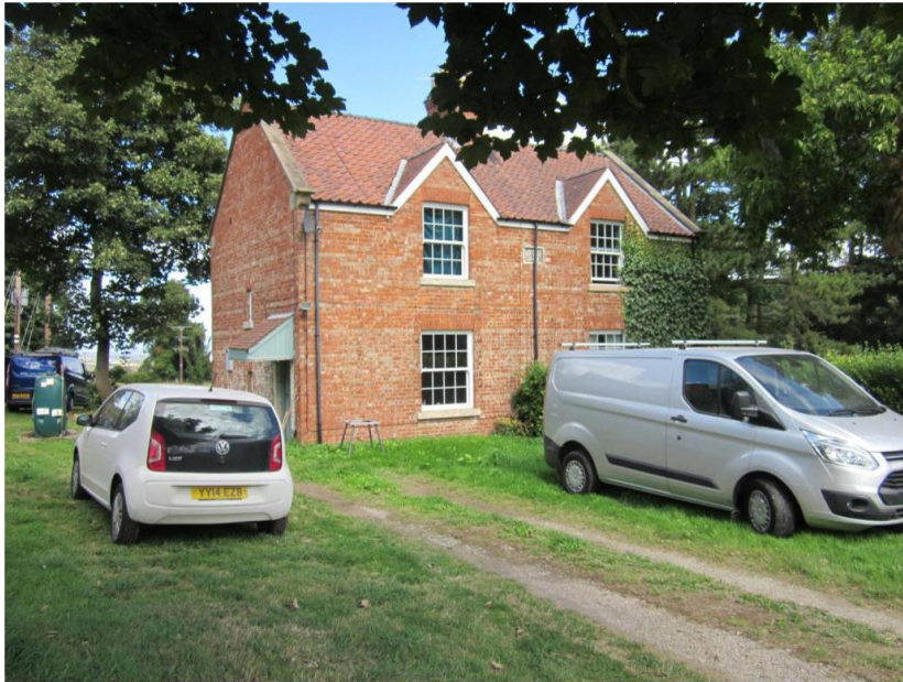
Fig 8 Building 2 Anna Cottages
