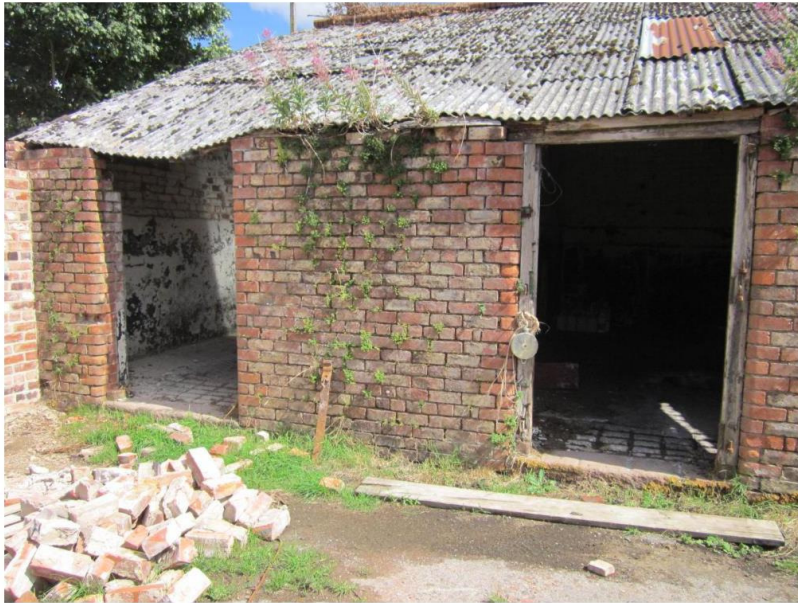
Fig 22 Building 6 West elevation
