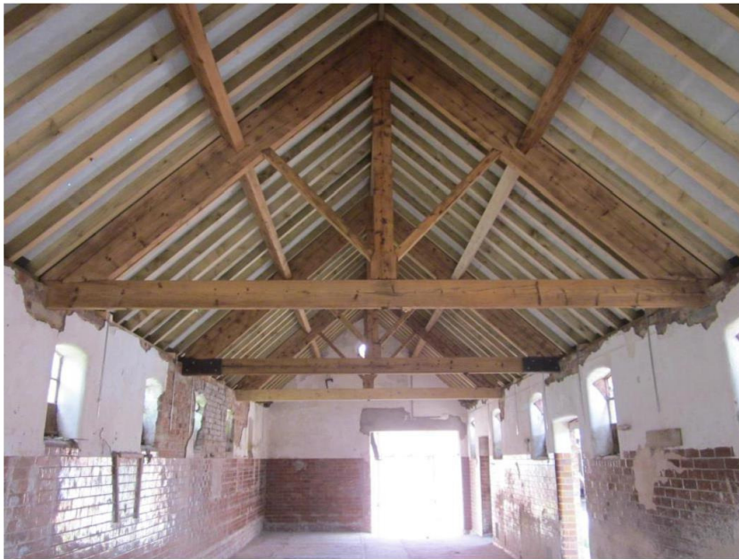
Fig 11 Building 3 Roof structure
