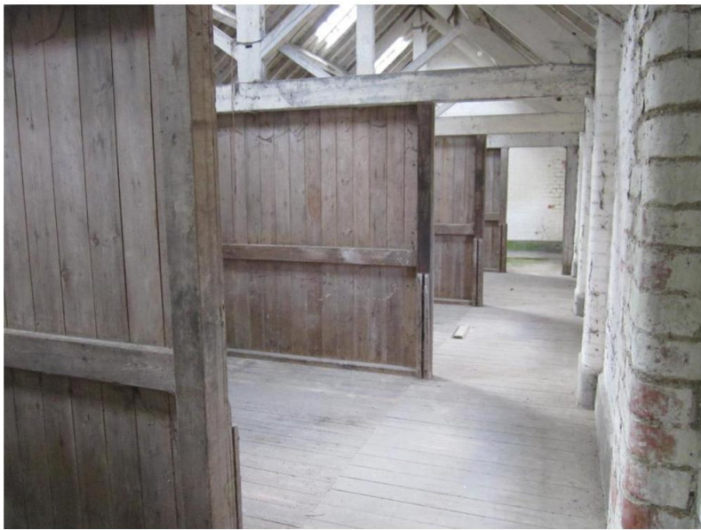
Fig 19 Building 4 First floor storage area
