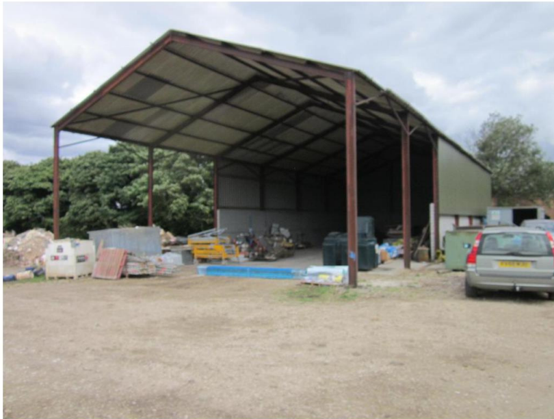
Fig 26 C20 steel-framed north-east shed
