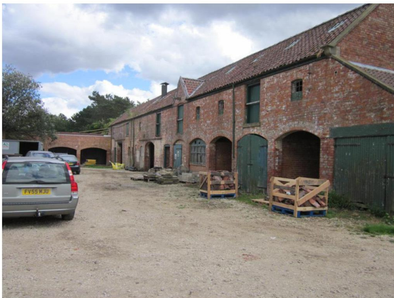
Fig 13 Building 4 North elevation
