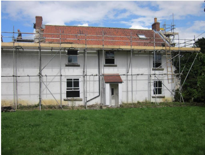
Fig 6 Building 1 South elevation
