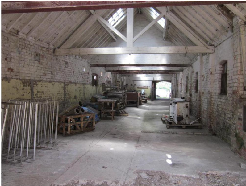
Fig 16 Building 4 West range interior
