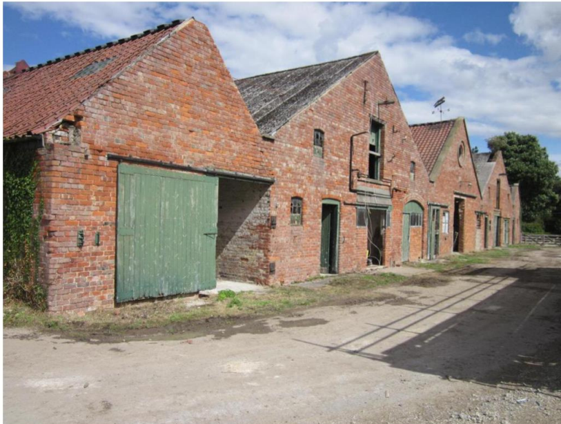
Fig 12 Building 4 South elevation
