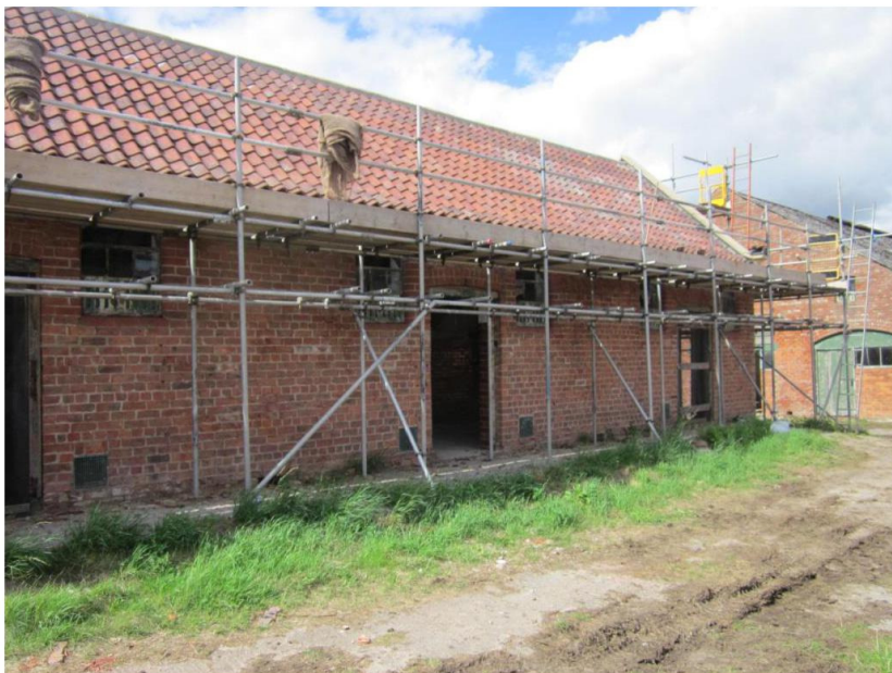
Fig 9 Building 3 East elevation
