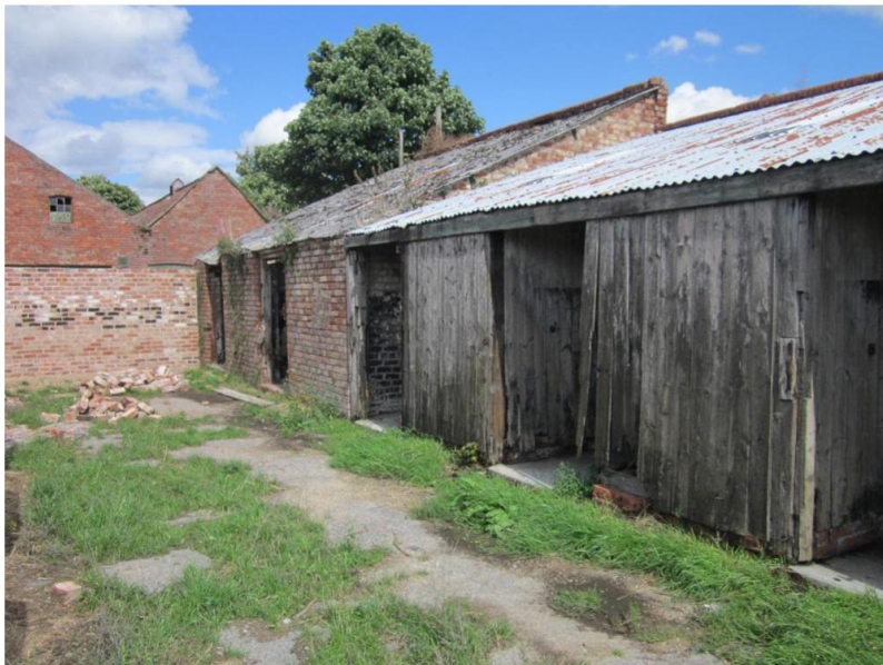
Fig 23 Building 6 and timber sheds to south
