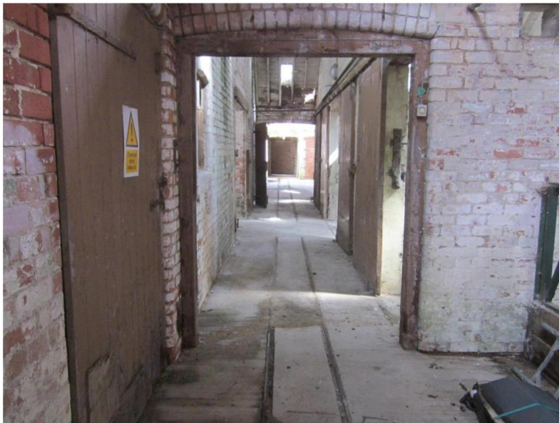
Fig 17 Building 4 Railway track to south of north range
