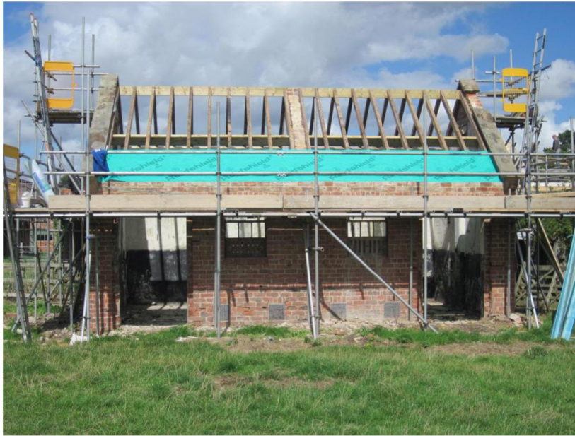
Fig 24 Building 7 South elevation
